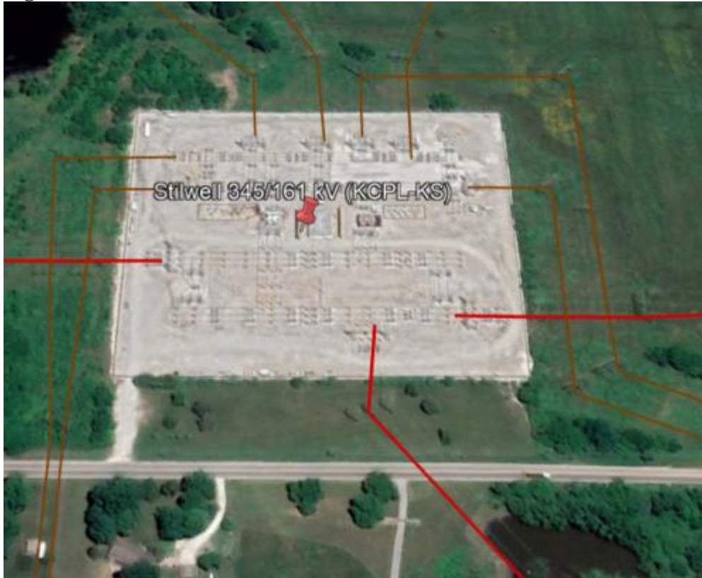
Figure 28 – Stilwell 345 kV substation
